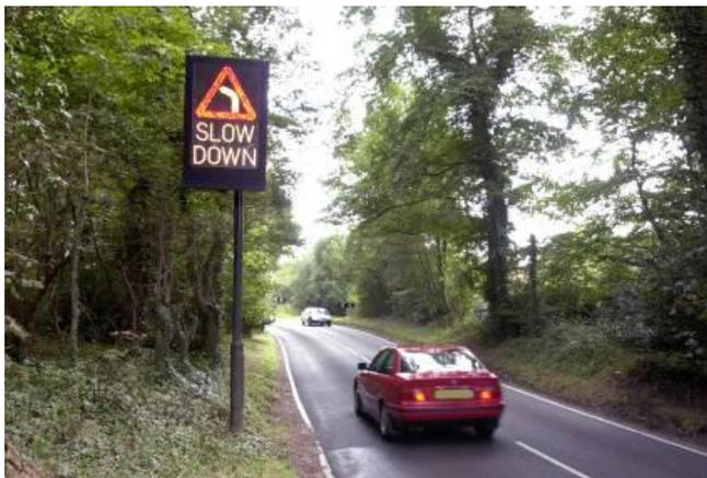
Figure 6: Vehicle activated curve/bend warning sign (driving on the left)
